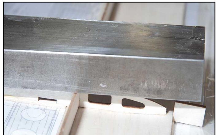
Figure 17: Plywood Bottom Sheeting Supports
